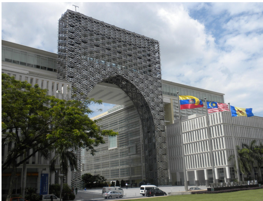
Figure 7: PJC office building
