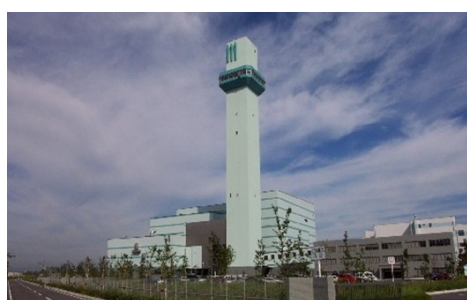
Figure 38: Thermal treatment facility (Picture of Eastern Clean Centre, Okayama, Japan)
