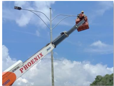
LED street light retrofitting project.
