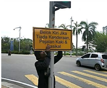
Maintenance on safety features for pedestrian walkway and bike lanes.
