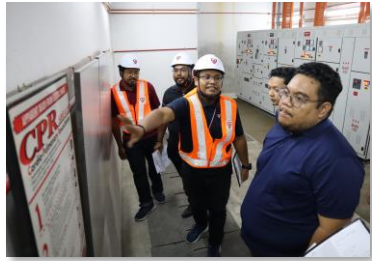
Building Energy Management Clinics.
