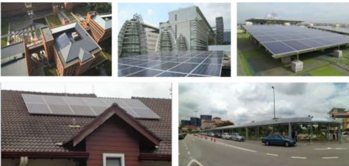
Photo 1: The use of photovoltaic (PV) and solar thermal systems on building in Putrajaya Source: https://www.ppj.gov.my
