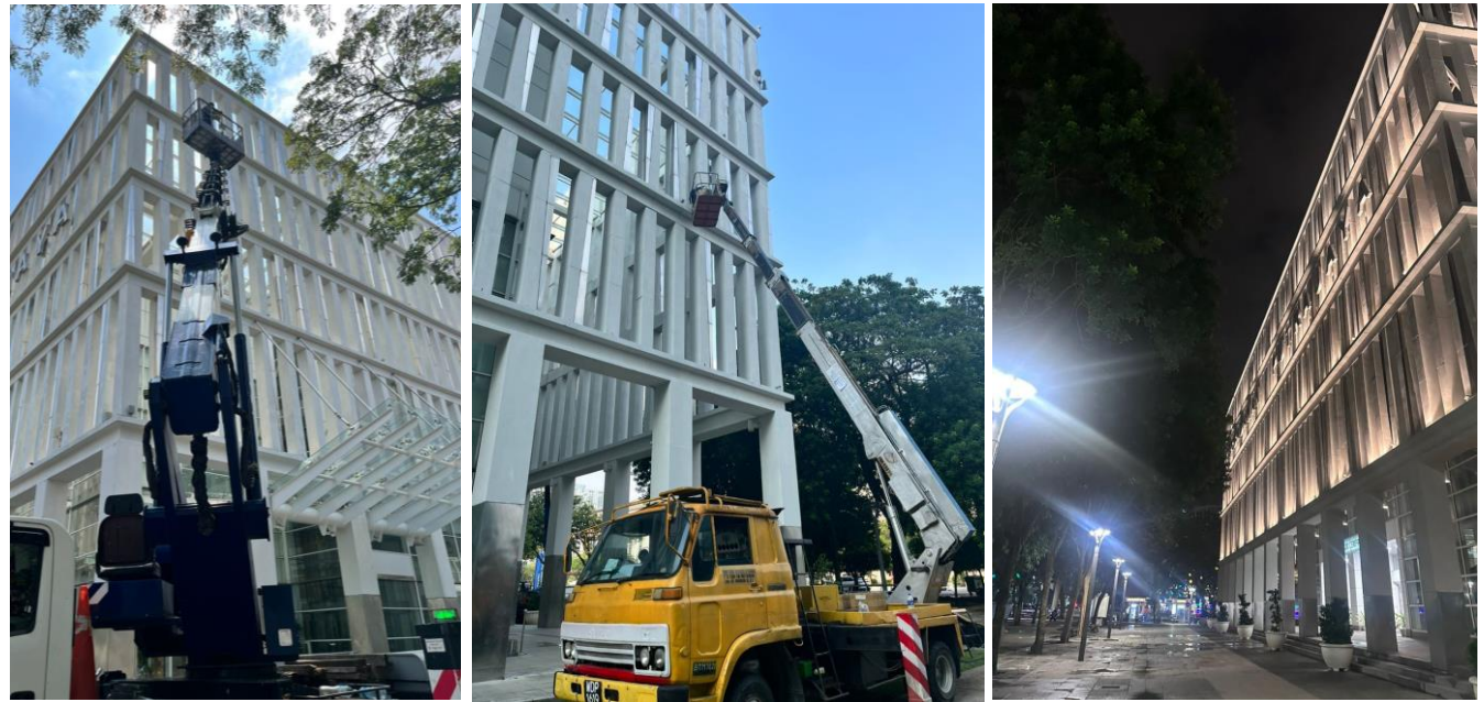
Screen Wall at the Conference Hall, Putrajaya Corporation Complex
