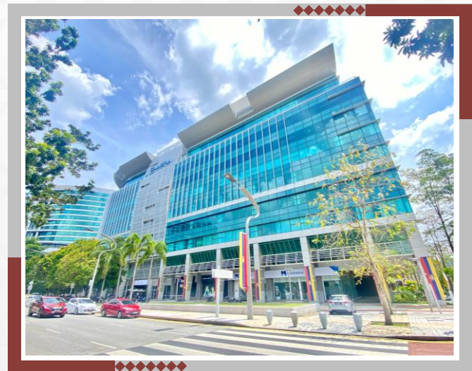
Galeria PjH, Precinct 4 (GreenPASS -Certified)
