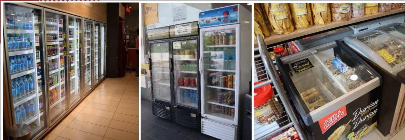
Chillers and freezers operating 24 hours are among the main electrical equipment contributing to energy consumption in the operation of this premise, and these appliances does not have energy efficiency label. It is encouraged to adjust the temperature to the optimum level and to use 5-star energy-efficient appliances to save on utility bill costs.
