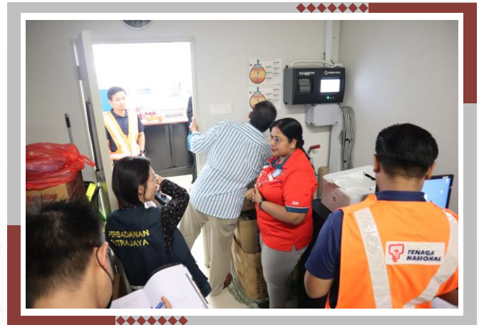
Walk through the building was conducted to inspect electrical equipment and assess the level of energy efficiency.
